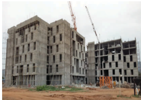
▲ Status of construction as on Mar 2019
